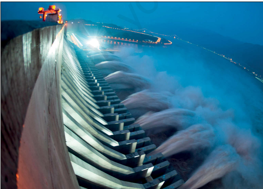
Figure 8.9 The Three Gorges Dam spanning the Yangtze River in Hubei province in China.
